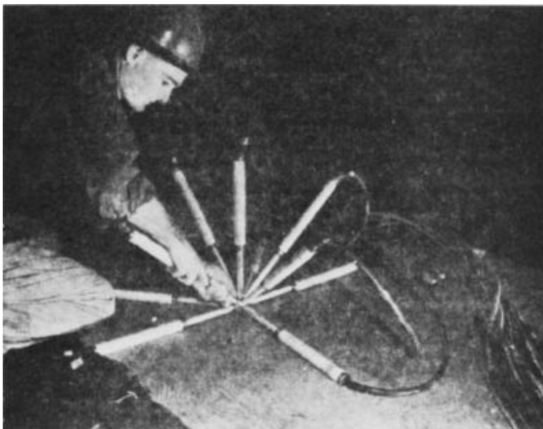
Figure C-3. Strain Meters Mounted on Spider (courtesy of the Bureau of Reclamation).
