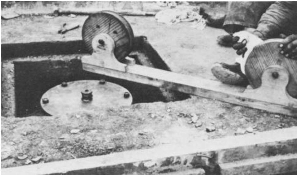
Figure 4-3. Lowering Plumb Bob Cap and Wire Through Suspension Plate (Courtesy of the Tennessee Valley Authority).
