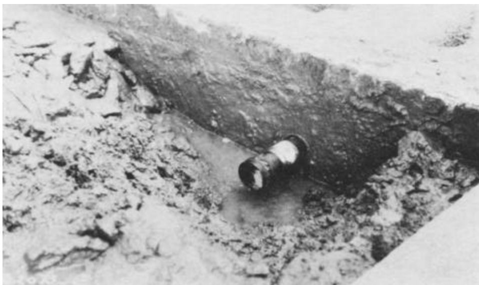
Figure C-12. Joint Meter Socket in Place (Courtesy of the Tennessee Valley Authority).
