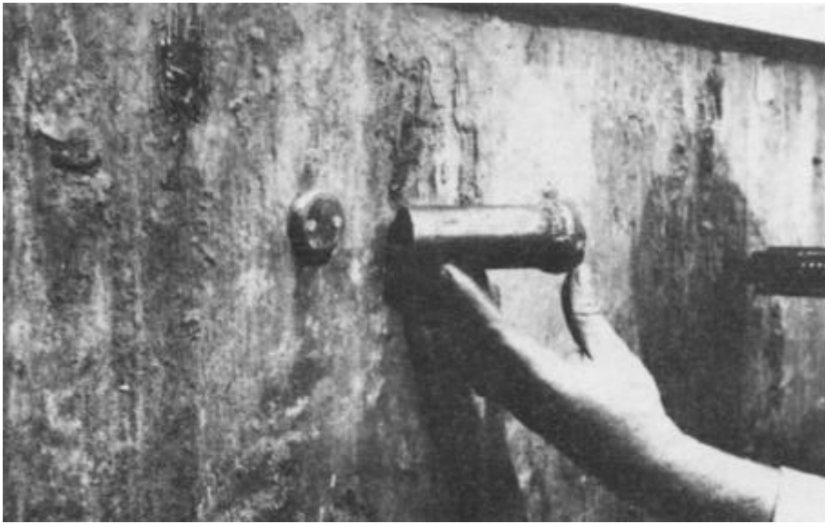
Figure C-10. Joint Meter Socket Plug (Courtesy of the Tennessee Valley Authority).
